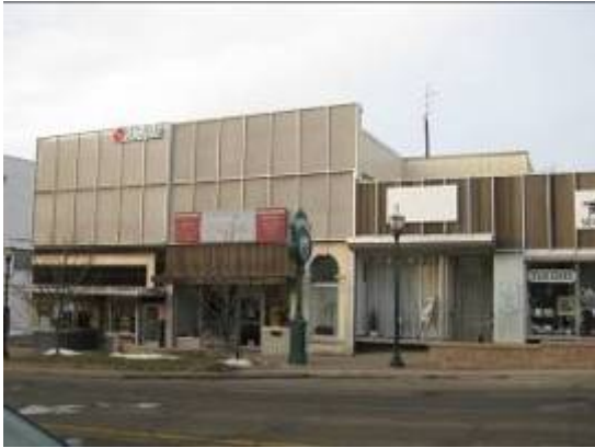
Last Un-restored Building Façade
